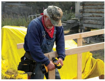
Mennonite Disaster Service volunteer Amos Diener drills a handrail on a new handicap ramp for a home damaged by flood waters at Stevens Village, Alaska. The handicap ramp became necessary because Amos and his fellow volunteer raised the house two feet to prevent future flood damage. Photo: FEMA/Ben Brennan
