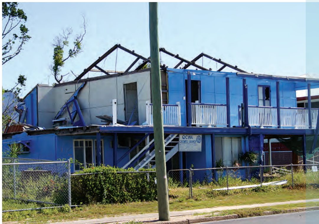
The Country Women's Association hall in Cardwell remains damaged.
