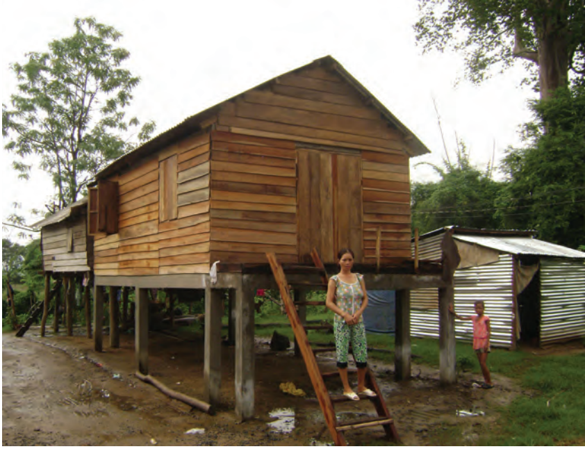
The new houses on stilts effectively resist next disasters and highly respond to local contexts.
