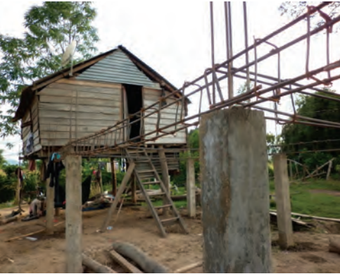
Based on an in-depth understanding of local context, together with community consultation, Tran Tuan Anh and Nguyen Quoc Thang came up with the final design with the utilisation of reinforced concrete for skeleton and timber for covering in the traditional typology of housing on stilts.
