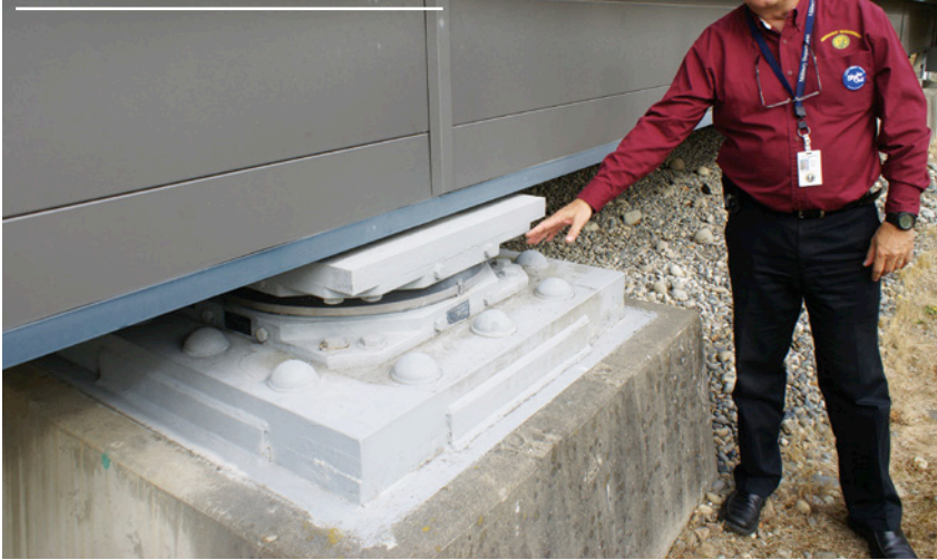
Chris Utzinger points to the earthquake resistant piles the Washington EOC is built on. The building will move as though it was on water.
