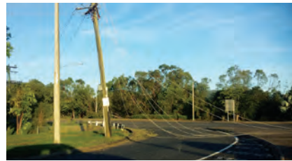
Some of the lesser damage on the way into Rocky.
