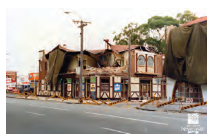
Damage to the Parkview Hotel, Maitland Road, Islington (source: The City of Newcastle).
