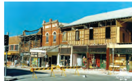
Union Street shops sustained severe damage (source: The City of Newcastle).
