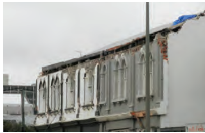
Extensive parapet damage in Christchurch (source: Risk Frontiers).
