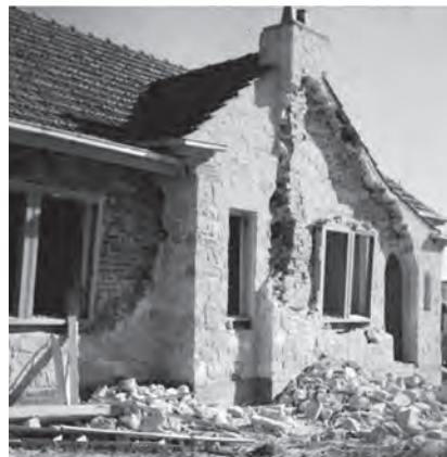
Heavily damaged house in Seacombe Park (source: Government of South Australia. Department of State Development).
