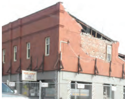
Facade collapse (source: Risk Frontiers).
