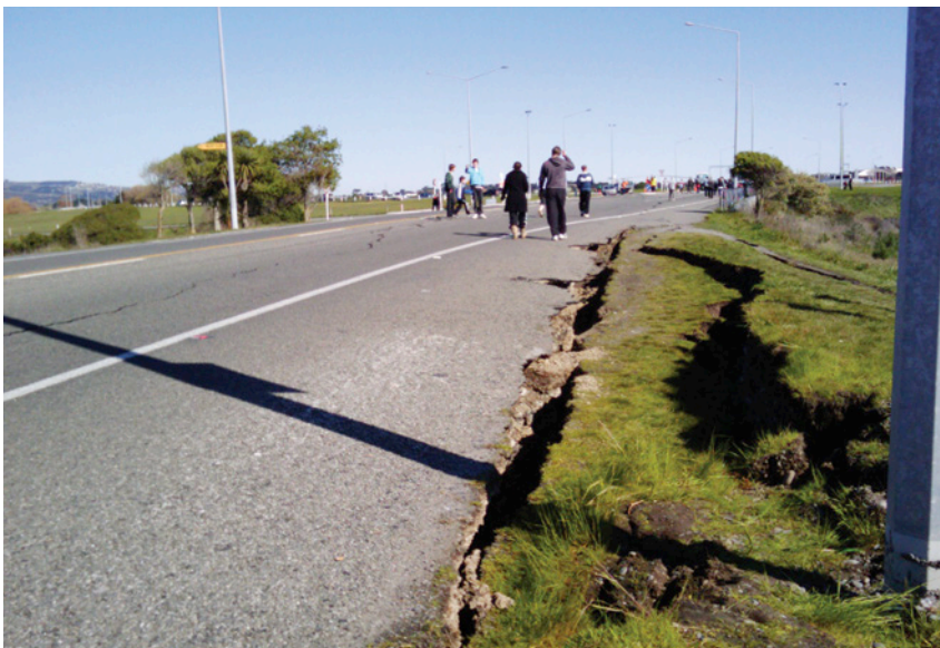
Christchurch earthquake, 2010. Photo by Richard Walker.
