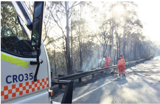
Cronulla 35 conducting road clearing operations on Heathcote Road.
