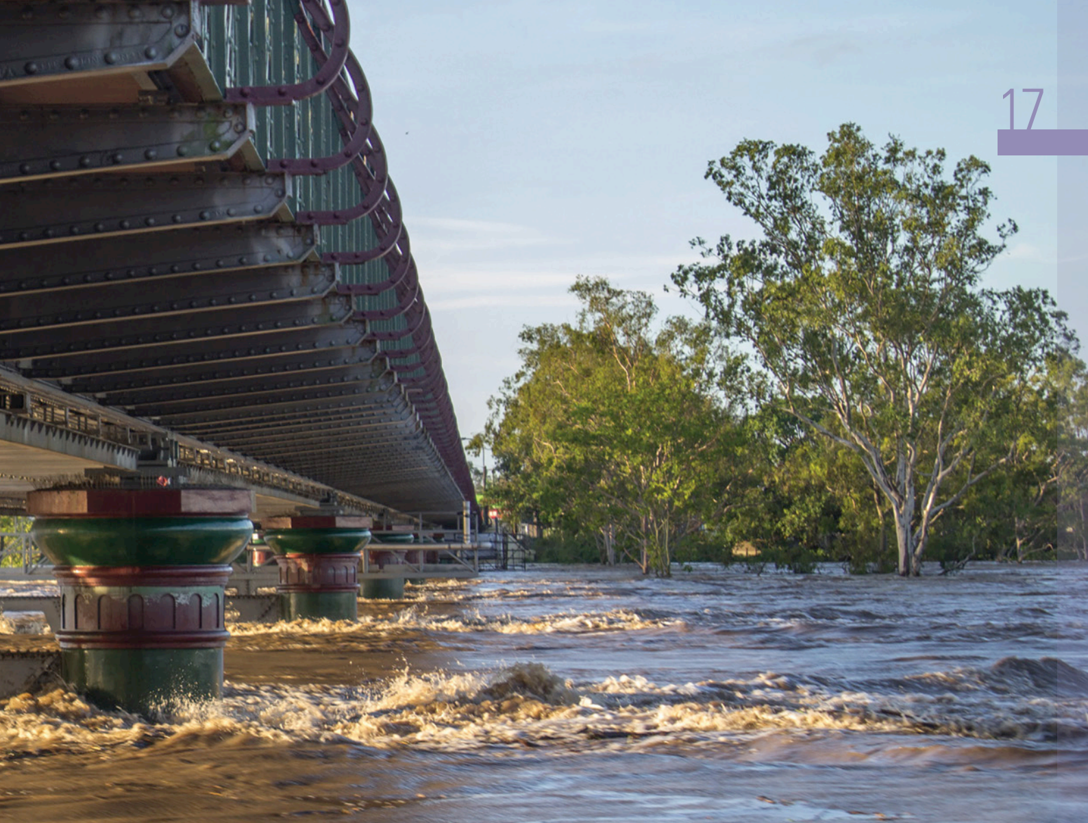
Rising water. View from the southern end (right bank) of the Burnett Traffic Bridge over the Burnett River, Bundaberg, 2012. Photo source: Flickr, All Creative Commons.
