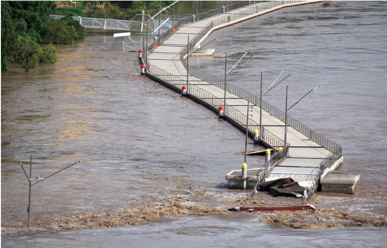
The Riverwalk between the Story Bridge and New Farm is torn apart by 4.2m flood waters. In the early hours of 13 January 2011, part of the 850m walkway broke off, and had to be carefully steered by tugboat between the Gateway Bridge supports to avoid a collision. Photo by Stephenk1977, Flickr, All Creative Commons.
