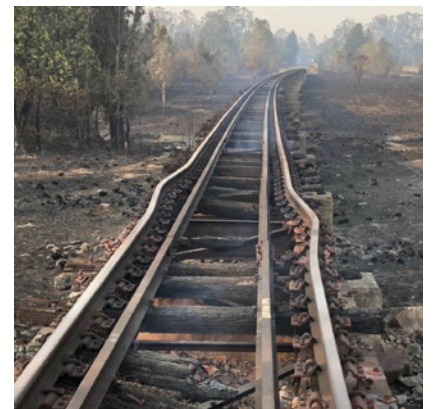
Part of the North Coast line damaged in fires. Picture: Facebook.
