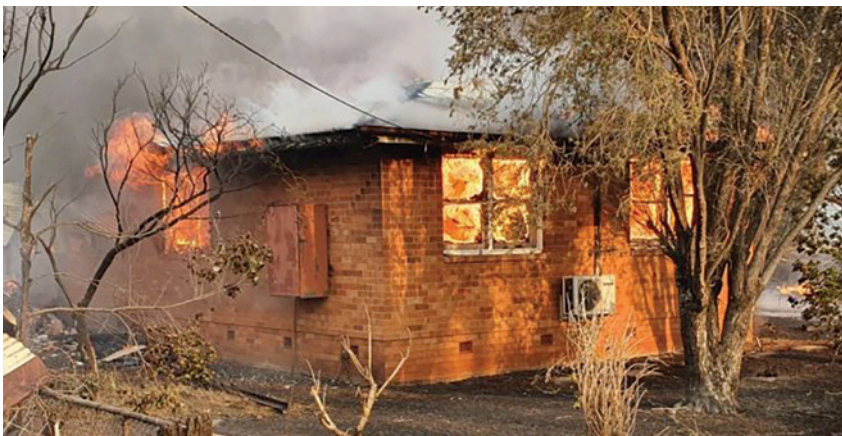
This house in Rappville was gutted by the fire. ABC News: Matt Coble
