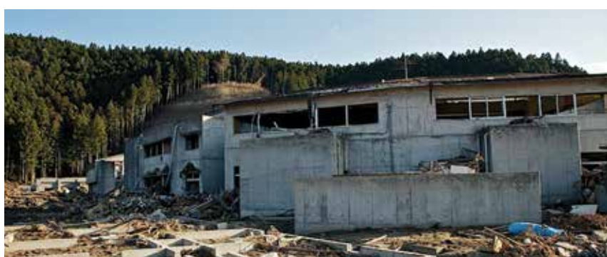
Okawa Elementary School that was devastated by the tsunami. Note the hill immediately behind the school where the children could have easily evacuated to for safety. It would have taken the group less than five minutes to climb to the top of the hill. Image credit; Carsten Knoche. Reproduced from Flickr 2011. https://www.flickr.com/photos/carstenknoche/5876774520/in/photostream/
